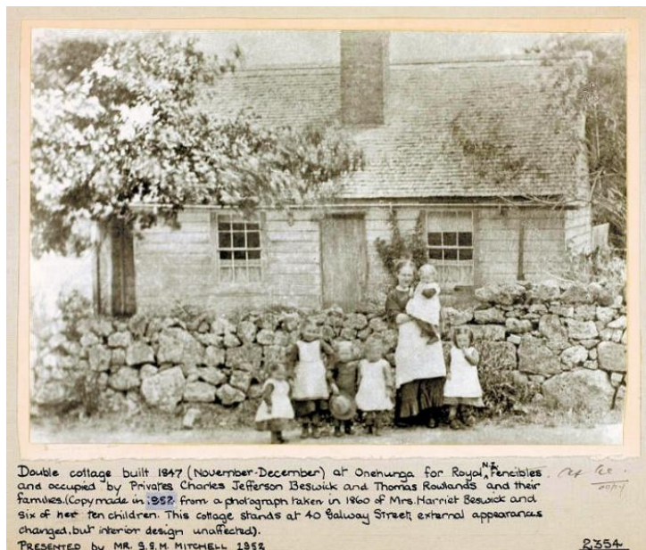
This early photo of Charles Beswick's Fencible Cottage at 40 Galway Street, Onehunga (formerly Albert Street)—now at Howick Historical Village—is not accurately described, as the children could not all have been Harriet Beswick's. See: https://www.rter.co.nz/onehunga.html
